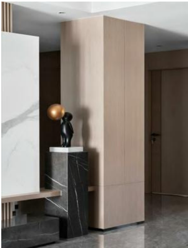
Effect of PVC wall panel slotting to wrap columns
